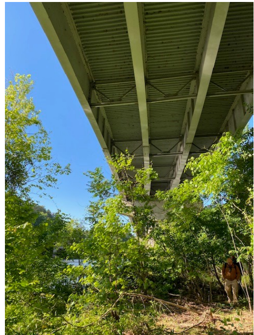
I-26 over gateway corridor
